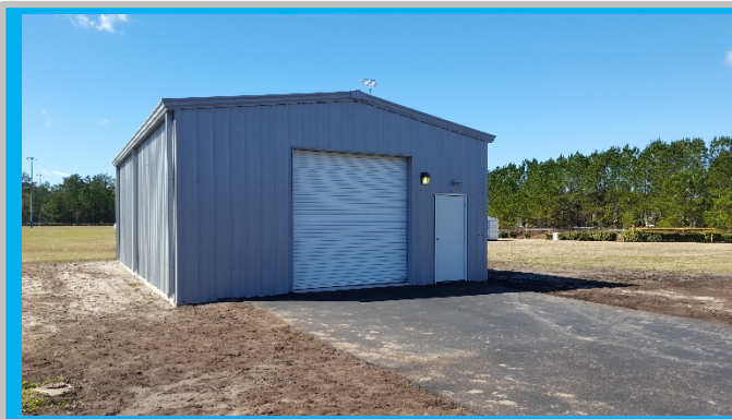
St. James High Athletic Storage – Completed
