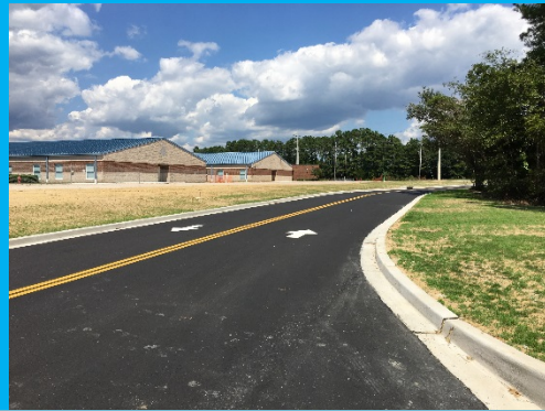
NMBM – Pavement/Curb & Gutter Now Complete
