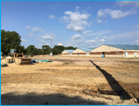
NMBM – Building Pad Graded for Foundation
