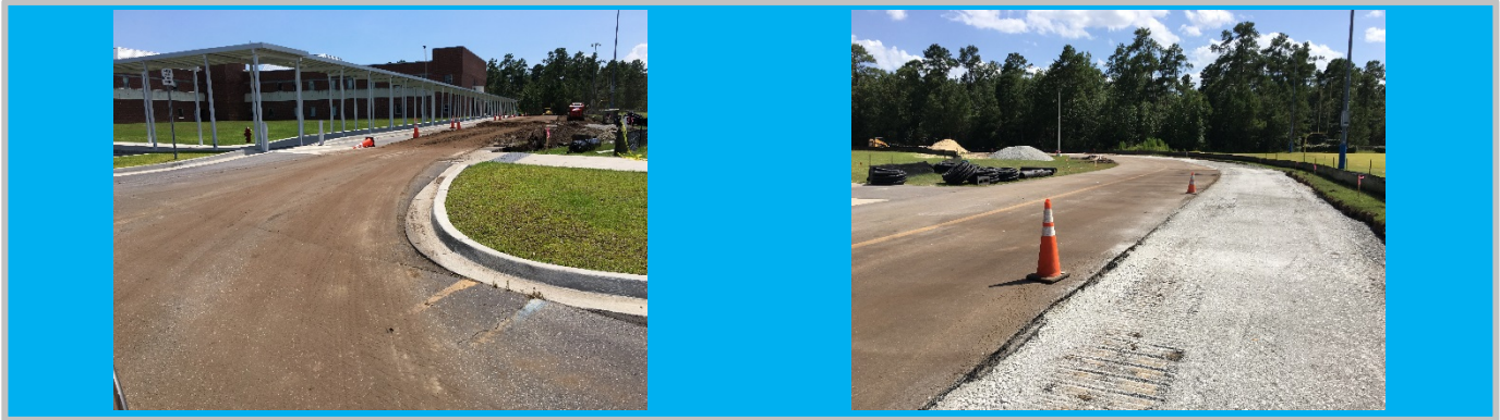
BEFORE - Begin Loop Widening
