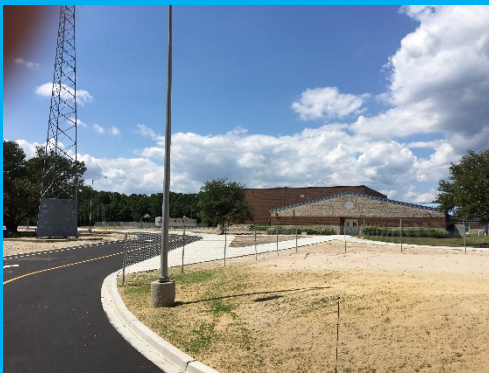
NMBM – New Asphalt Pavement @ Bus Loop
