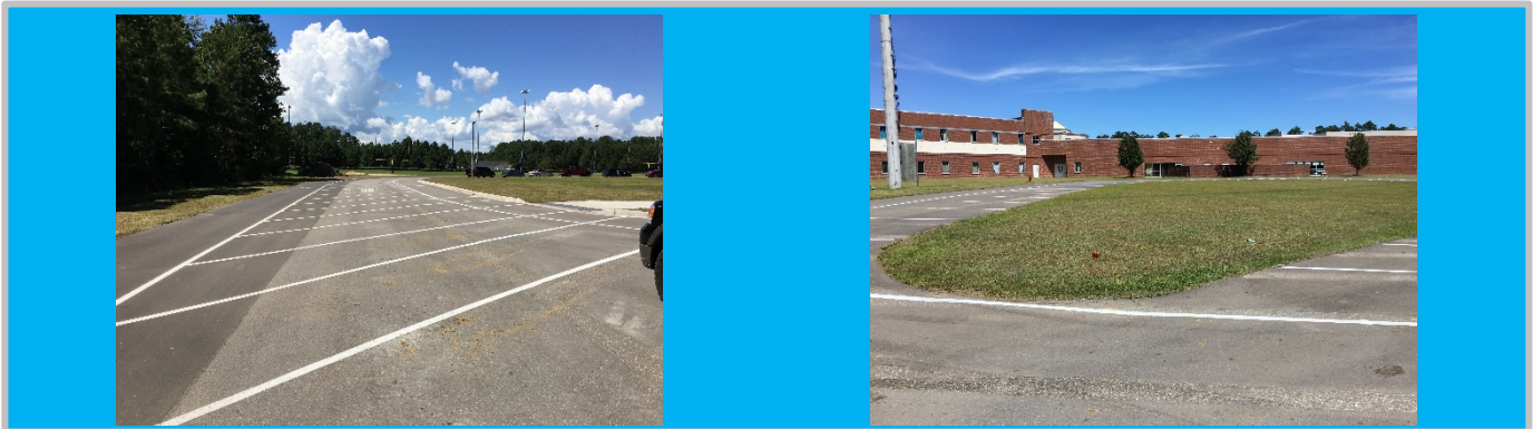
AFTER - Striped so that 20' Emergency Lane Maintained
