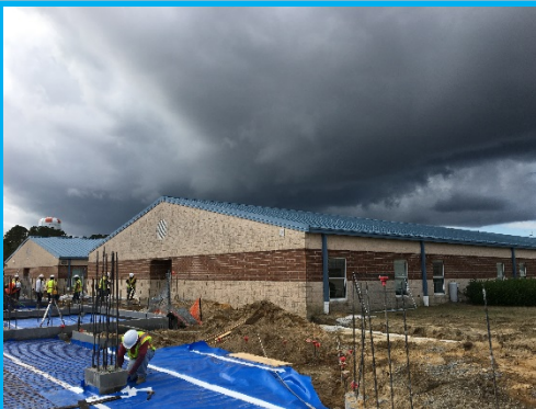
Slab on Grade Construction 80% Done
