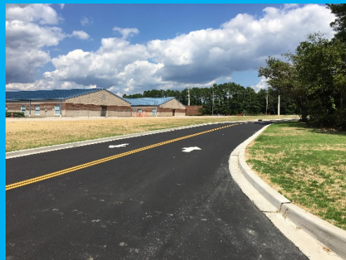
Pavement/Curb & Gutter Now Complete
