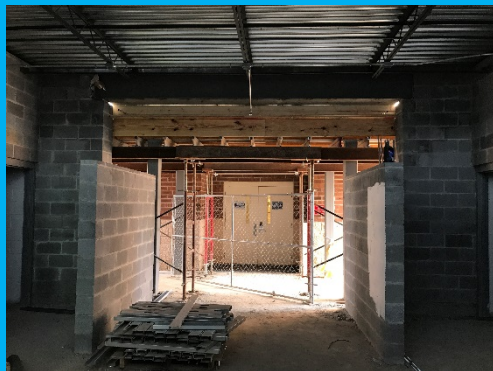
Connections to Existing Building Ongoing
