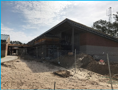
Steel Erection & Masonry Nearly Completed
