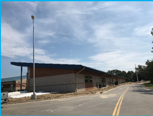
Roof and Exterior Metalwork
