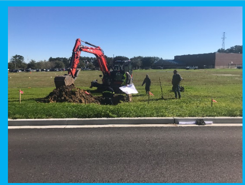
Utility Locates Under Soccer Field
