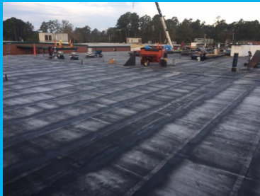
Non Functional Skylight Removal – SCES
