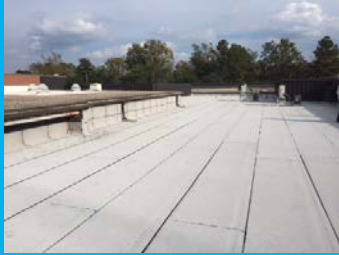
Completed Roof WPMS
