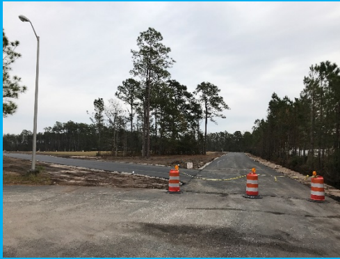
New Parent Loop Entry Location
