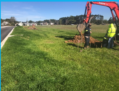
Utility Locates Under Soccer Field
