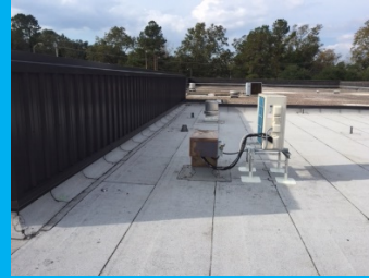
HVAC Upgrade WPMS
