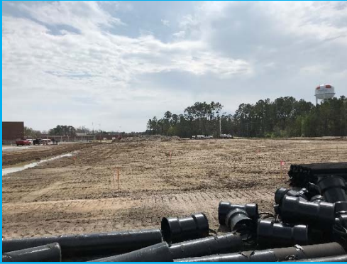
Entire Field – 1' Material Cut Out & Replace
