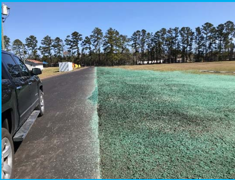
Road to back of SJE Completed
