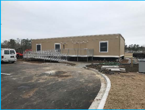
Bus Office Modular Installed
