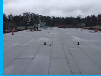
Roof Where Skylights Were Removed
