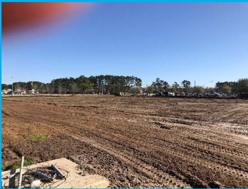
Field Footprint is Currently Dry and Work Ongoing
