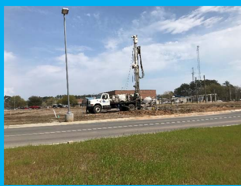
Well Driller is On Site & Working
