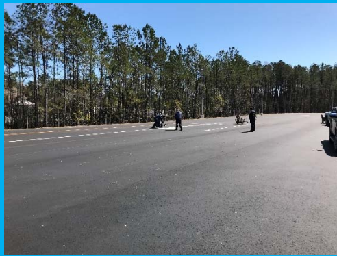
Bus Parking Lot Paved & Striped w/ Training Pad
