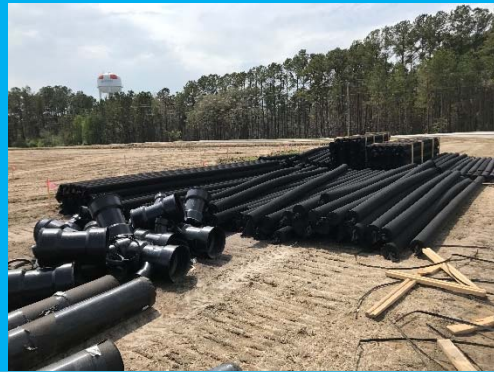
All Drainage Materials on Site
