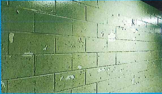
Corridors Prior to Stripping
