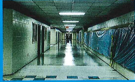
Corridors After Stripping & Painting
