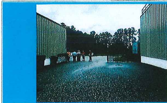
New Addition to DO Right Structure
