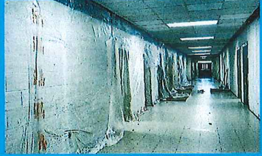
Corridors During Stripping Process
