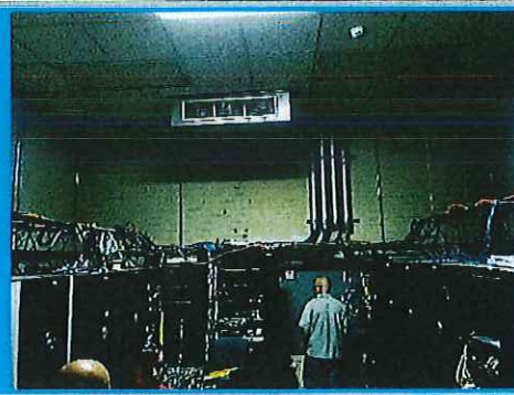
Inside DO Server Room - Far Wall to Penetrate for Ductwork
