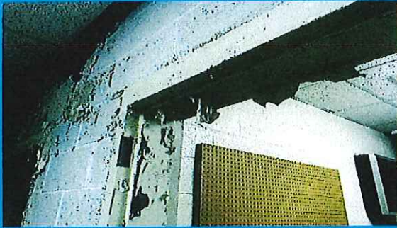
Walls/Door Frames After Stripper Applied
