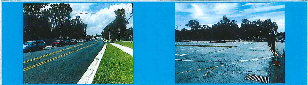
11 th Avenue Turn Lane @ Morning Drop Off
