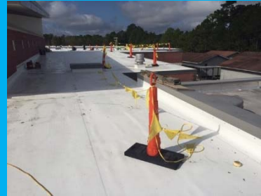
New Parapet Sheet Metal Cap
