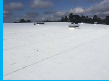
Educational Wing with Roof Vents
