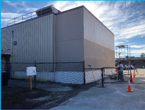
New Addition to DO C-Building
