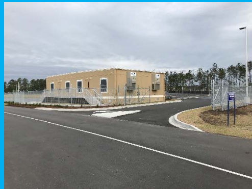
Bus Office @ Driver Entry
