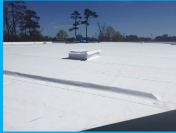
Gym Roof Completed
