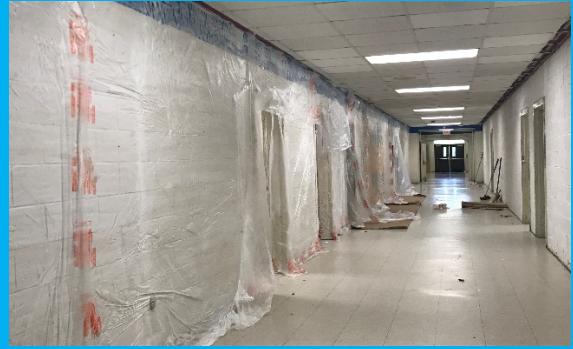
Corridors During Stripping Process (Example)
