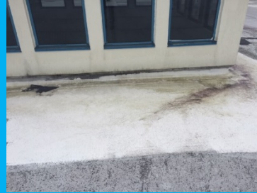
Skylight Area of Roof to be Modified
