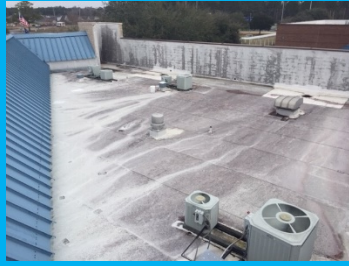
Existing TPO Roof
