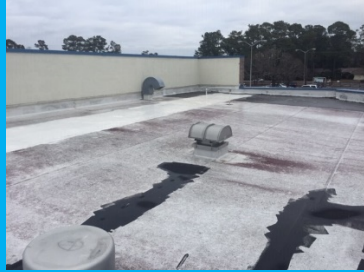
Existing TPO Roof
