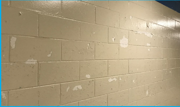
Corridors Prior to Stripping (Example)
