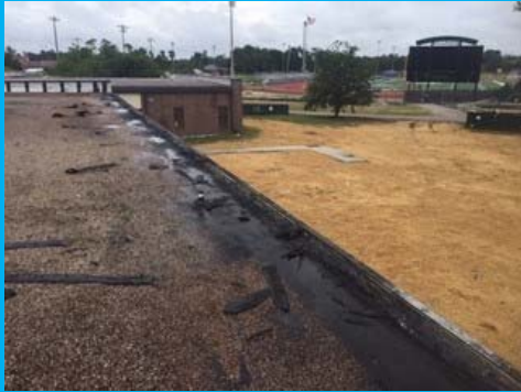
Prep Work for New Gravel Stop
