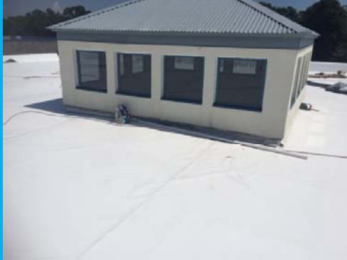
New TPO Roof Around Clerestory
