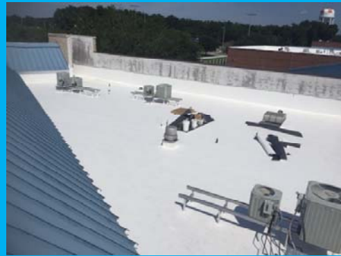
New HVAC stands
