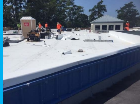
TPO Roof Membrane and Half Sheets
