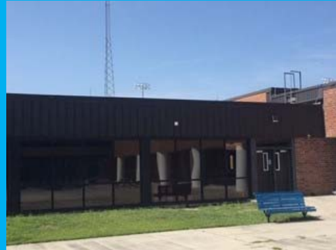
Courtyard Parapet Metal Coverings
