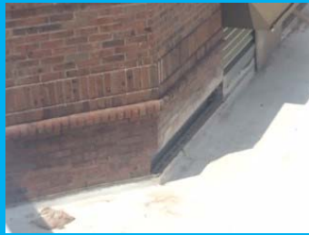
Through Wall Flashing Repair
