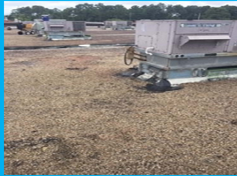
All Flashings around HVAC Curbs Repaired
