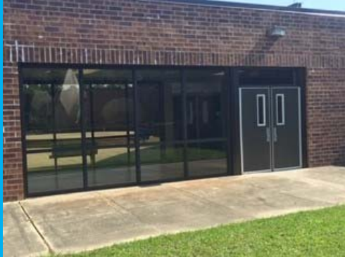
Portion of New Store Front
