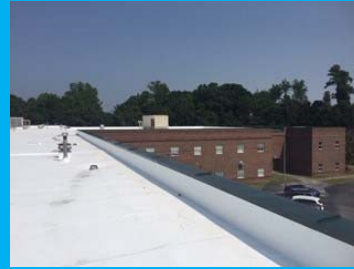
Completed TPO Roof and Parapet Cap
