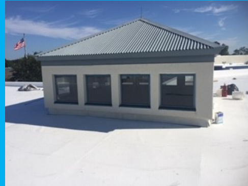
New TPO Flashings around Base of Clerestory
