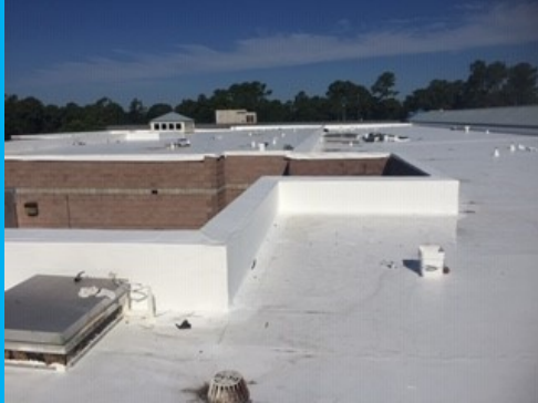
TPO Membrane before Parapet Cap
