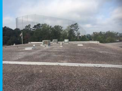
Coating of all Flashings and Control Joints
