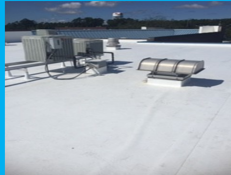
New HVAC Stands
