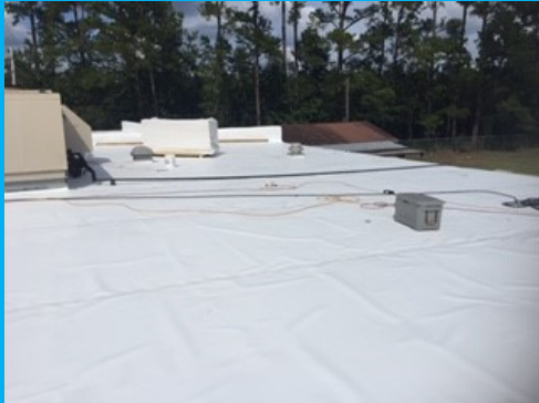
New 1.5" Cover Board and TPO
