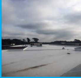
Completed TPO Membrane
