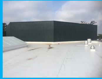
Metal Wall Panels Around Auditorium
