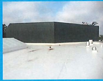
Metal Wall Panels Around Auditorium
