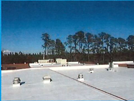
Finished TPO Roof
