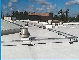
New Galvanized Piping
