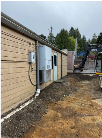
Storm and Sewer Exploration
