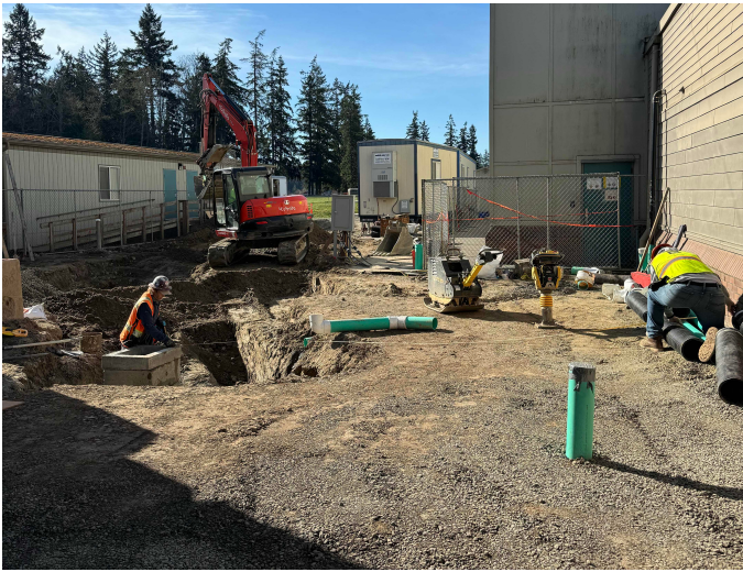
Sewer & Storm Installation
