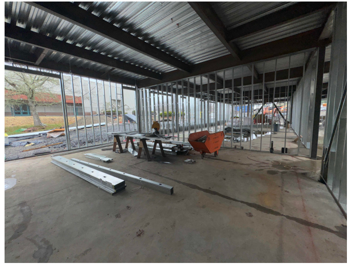
Start of 1st Floor Interior Metal Framing
