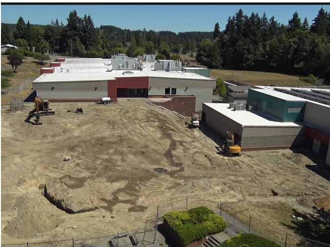
Start of Project
