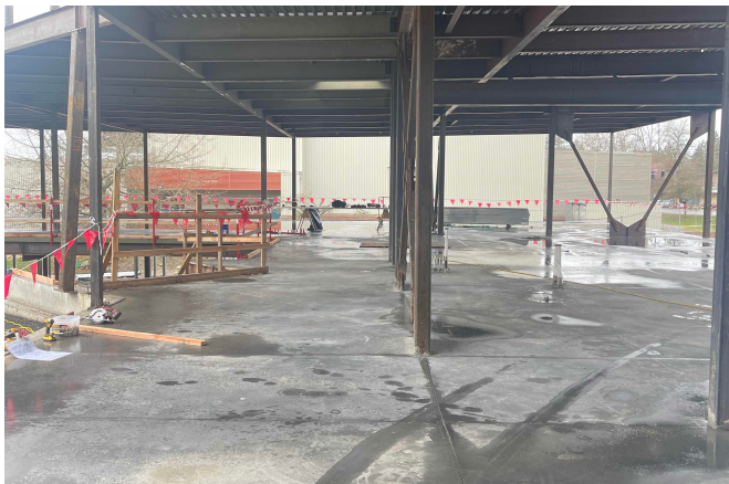
2nd Floor Concrete Completion
