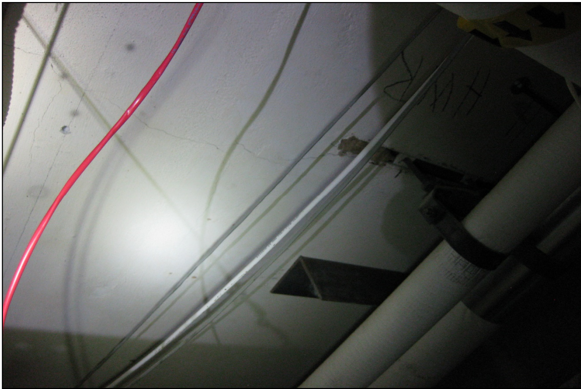
Photo 2: Cracking at Underside of 1 st Floor Corridor Slab
