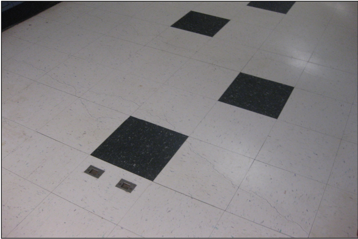
Photo 1: Typical Cracking in VCT Flooring at Southern End of 1 st Floor Corridor
