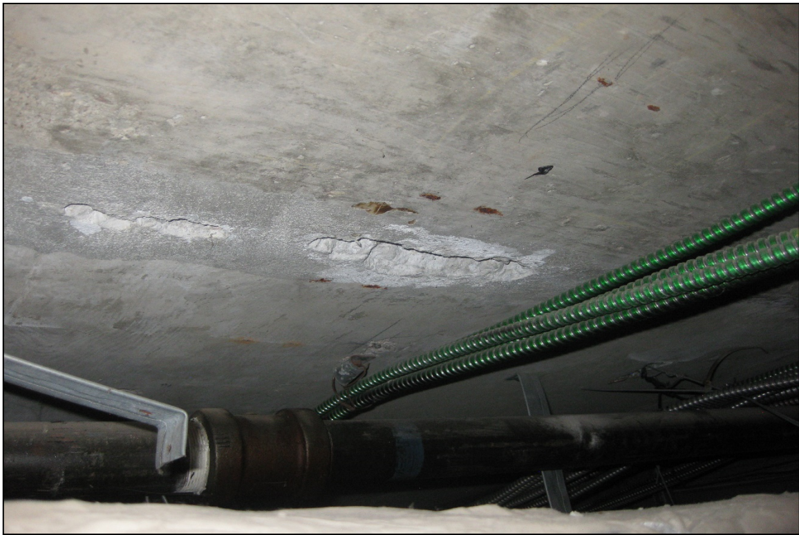
Photo 4: Exposed Rebar Chairs at Bottom of Concrete Slab
