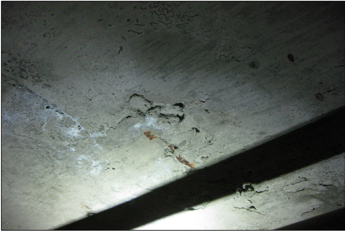
Photo 5: Mild Efflorescence and Exposed Rebar at Bottom of Concrete Slab
