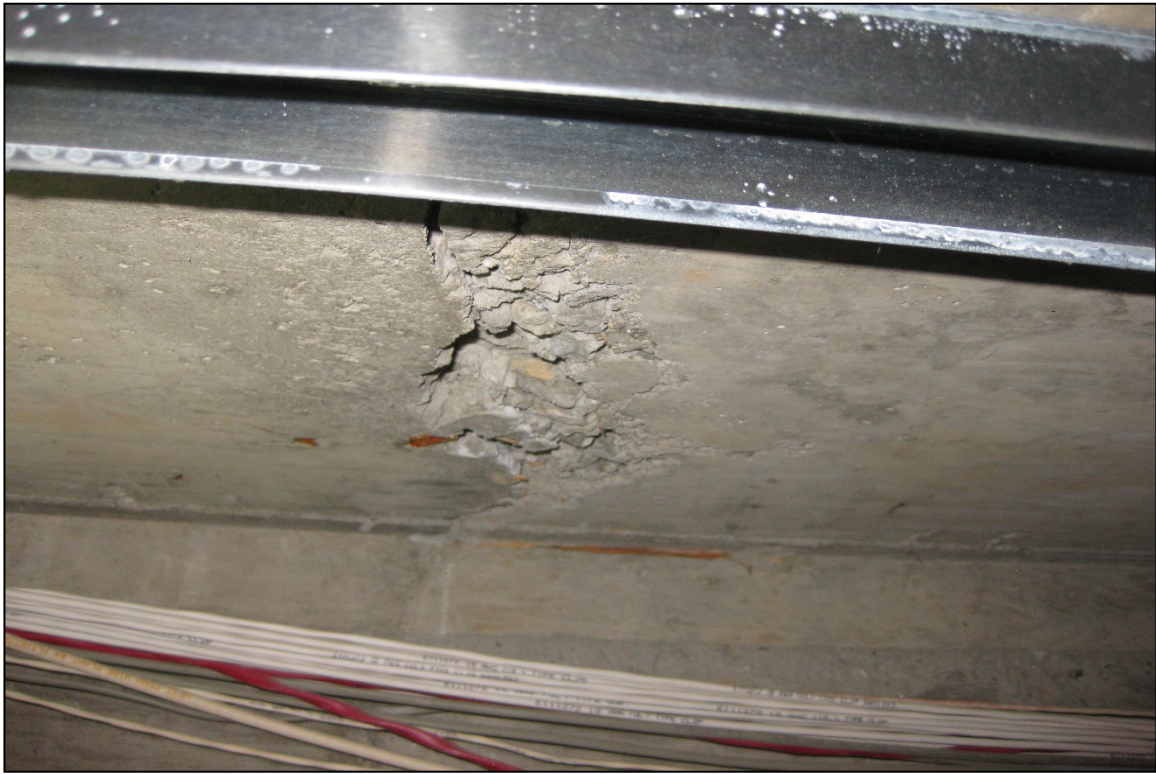
Photo 3: Typical Voids at Areas of Poor Consolidation
