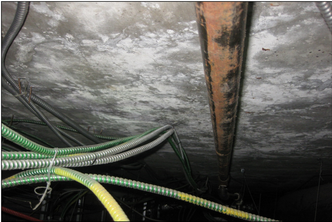
Photo 6: Previously Observed Significant Deterioration at Northern End of 2 nd Floor Corridor
