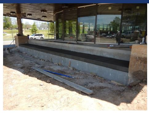
Micropile Reinforcement for New Canopy Columns
