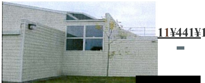
Cement plank clapboard is a new material that resembles traditional wooden siding with less maintenance.
