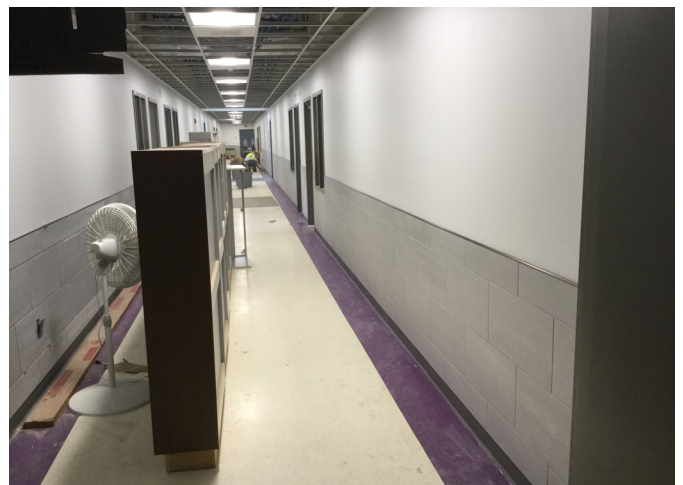
New Tile on Walls
