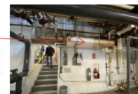
Looking north to stairs
