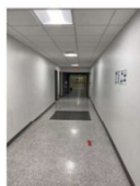
Access hatch in ES corridor
