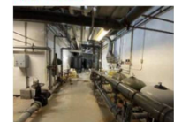
View south from stairs
