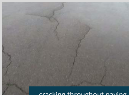
cracking throughout paving
