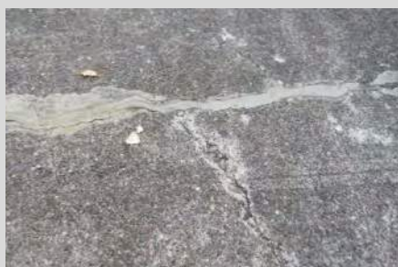
cracking paving
