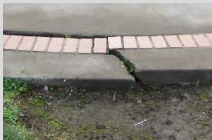
cracks in sidewalks
