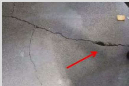
cracking on concrete floor
