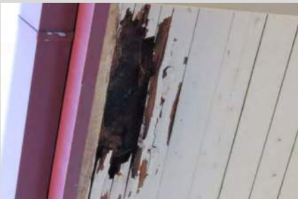
rotting roof soffits
