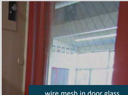
wire mesh in door glass
