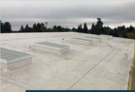
TPO roof condition
