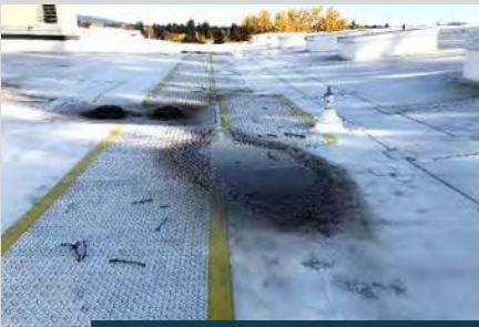
drainage issues on roof
