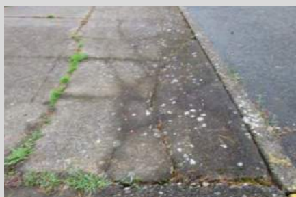
worn and cracked paving
