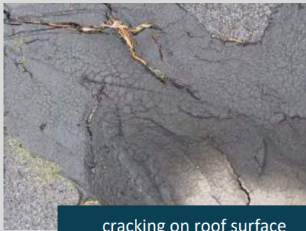
cracking on roof surface
