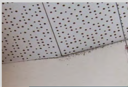
mold growth along ceiling
