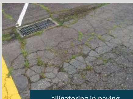
alligatoring in paving
