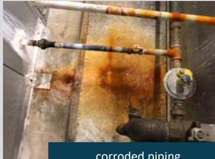
corroded piping
