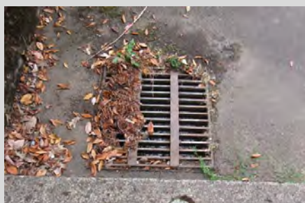
Clogged Storm Drains
