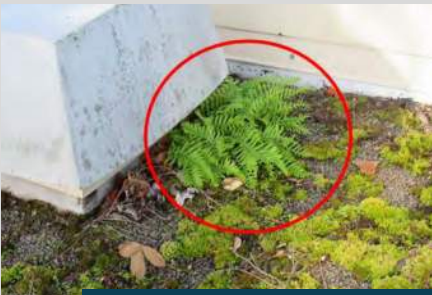
moss build up and drainage issues
