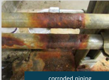
corroded piping
