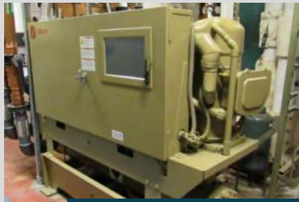
newly installed chiller
