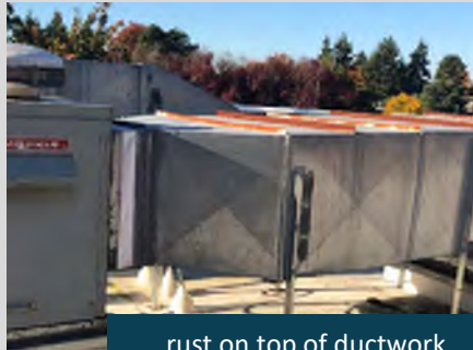
rust on top of ductwork
