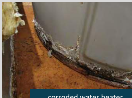
corroded water heater
