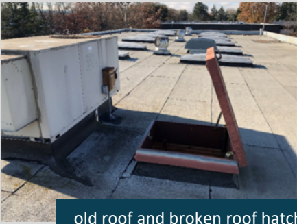
old roof and broken roof hatch
