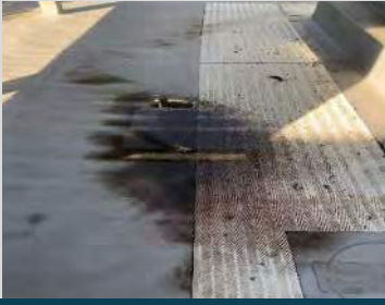
water not properly draining
