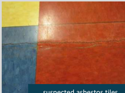
suspected asbestos tiles
