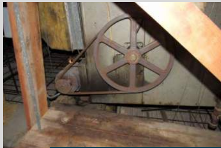
air handler missing belt guard
