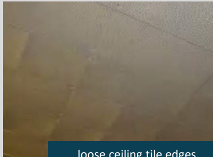
loose ceiling tile edges
