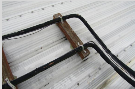
refrigeration lines insulation
