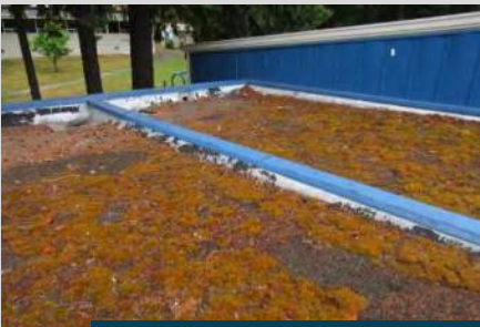
excessive moss growth on roof
