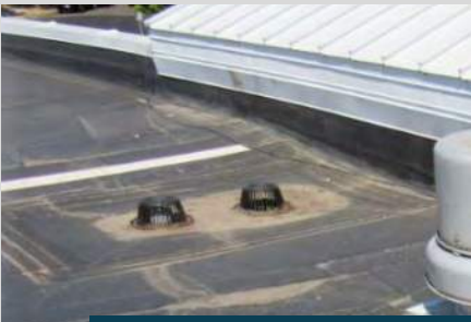
debris accumulated on roof
