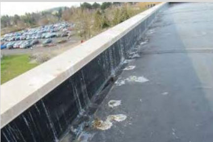
bird damage on exterior parapets
