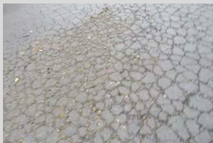
alligatoring on paving
