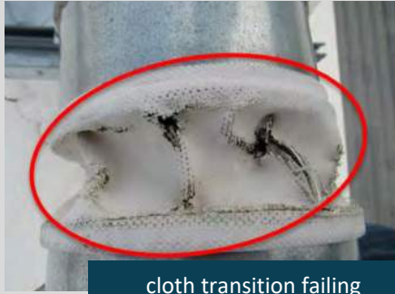
cloth transition failing
