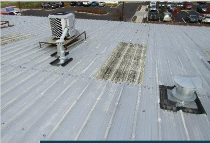
metal roof is worn
