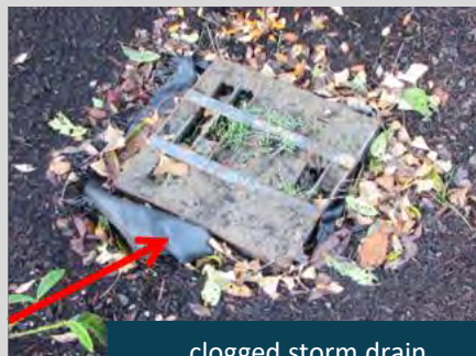
clogged storm drain
