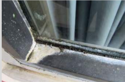
water intrusion at window
