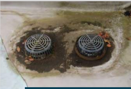
clogged roof drains
