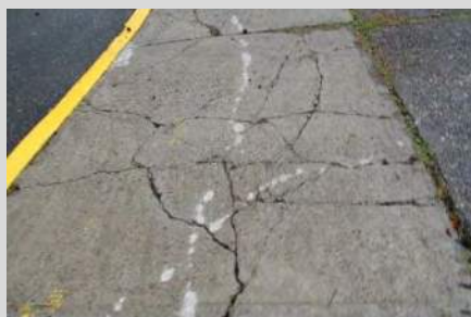
damaged pedestrian paving
