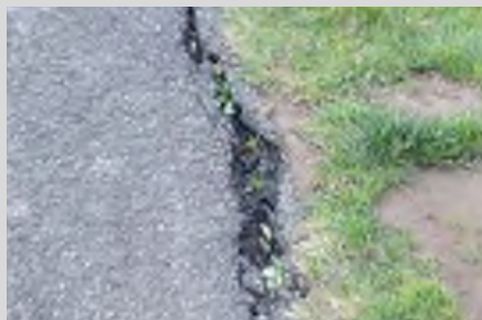
cracking and moss on paving
