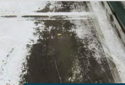
debris build up on roof
