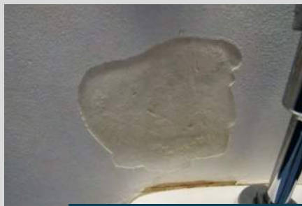
wall damage from plumbing leak
