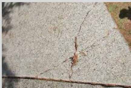
cracking on pedestrian paving
