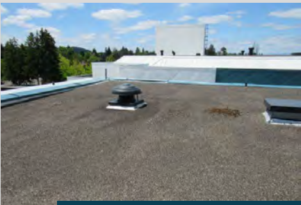
moss build up and drainage issues
