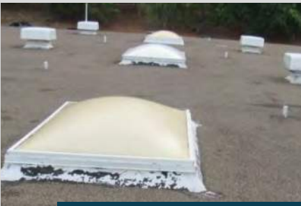
water intrusion at skylights
