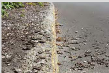
Damage to curb
