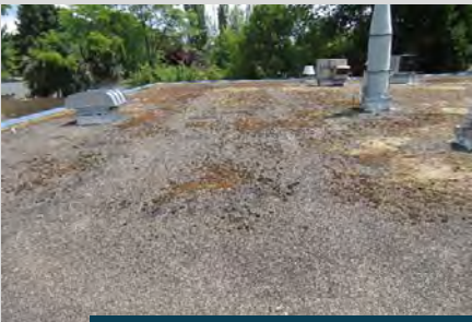
moss build up and bubbling
