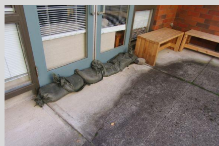
sand bags protecting from flooding
