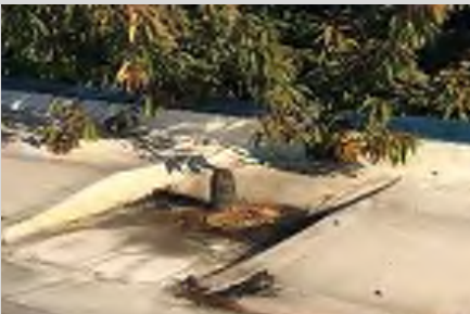
moss build up and drainage issues
