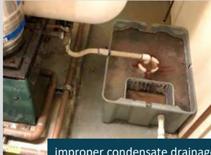
improper condensate drainage
