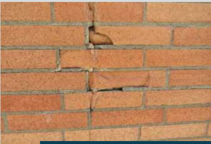
cracks in exterior brick
