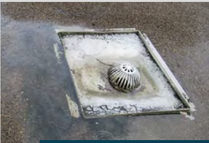
drainage issues on roof
