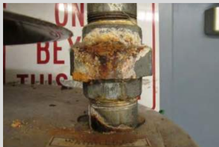
corroded plumbing equipment
