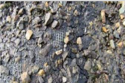
Roof exposed seams and bubbles
