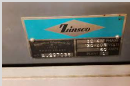
potential panel fire hazard
