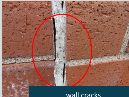
wall cracks
