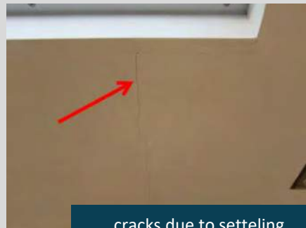
cracks due to settling
