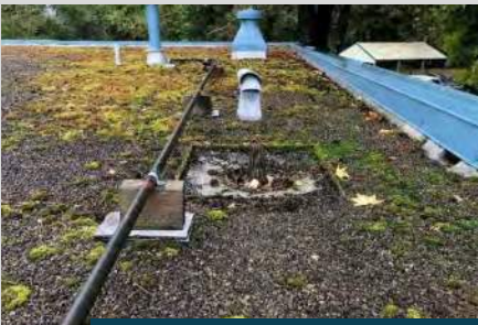
clogged drains and moss build up
