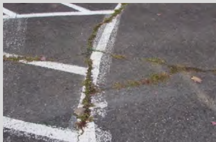
cracking on parking lots
