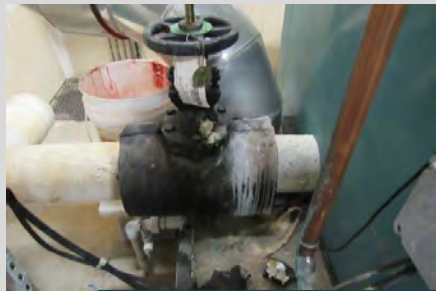
Leaking Valves
