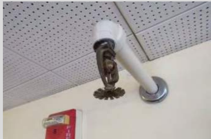
Aged fire sprinkler system
