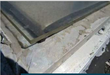
poorly sealed skylights
