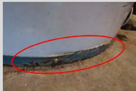
corroded hot water heater
