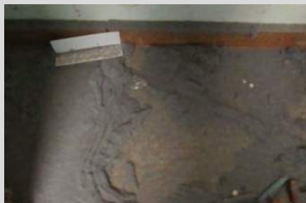
heavy dust at base of panels
