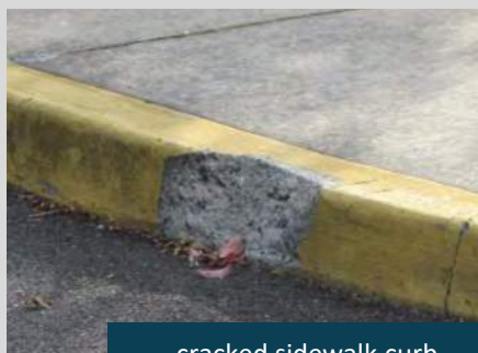
cracked sidewalk curb
