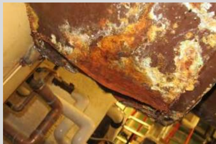
water heater burner tube
