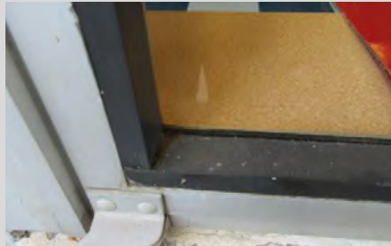
cracking along window
