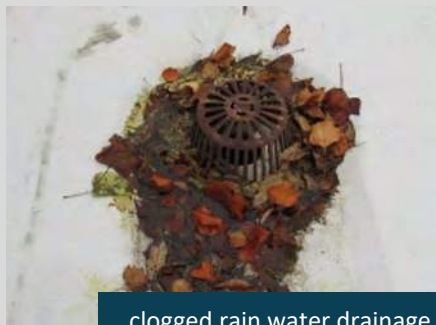
clogged rain water drainage
