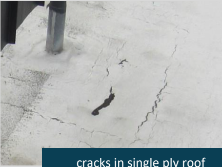
cracks in single ply roof
