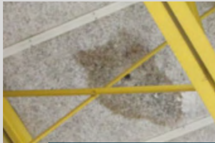
damage to gym ceiling
