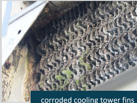
corroded cooling tower fins
