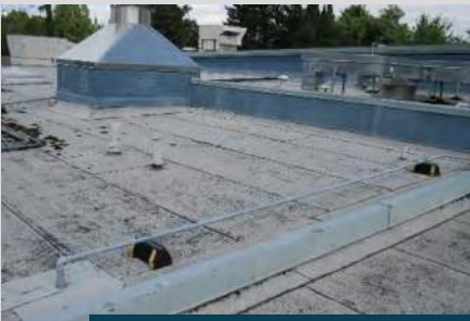
poor asphalt roof condition
