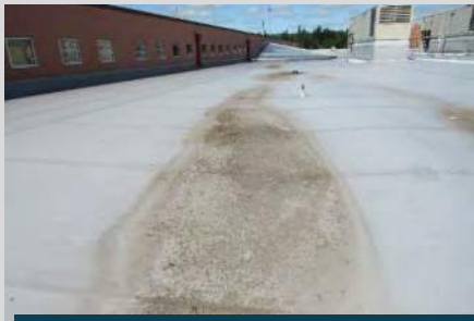
roof condition due to standing water
