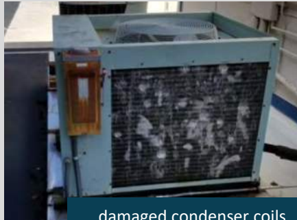
damaged condenser coils
