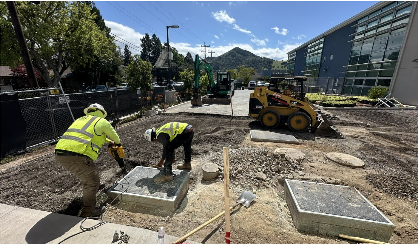
Base Rock Compaction at Receiving Area
