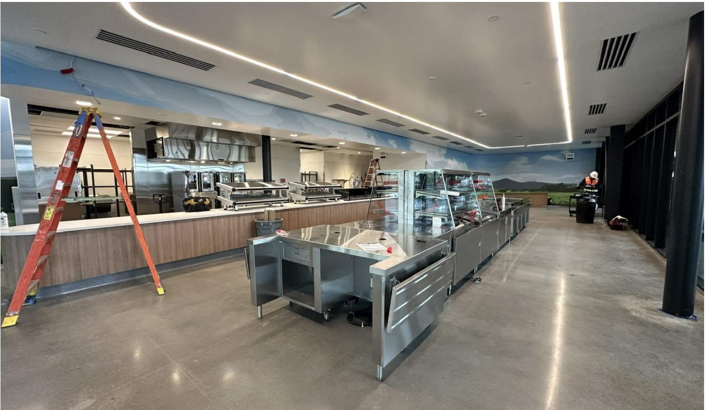
Track & Soffit Lighting Complete
