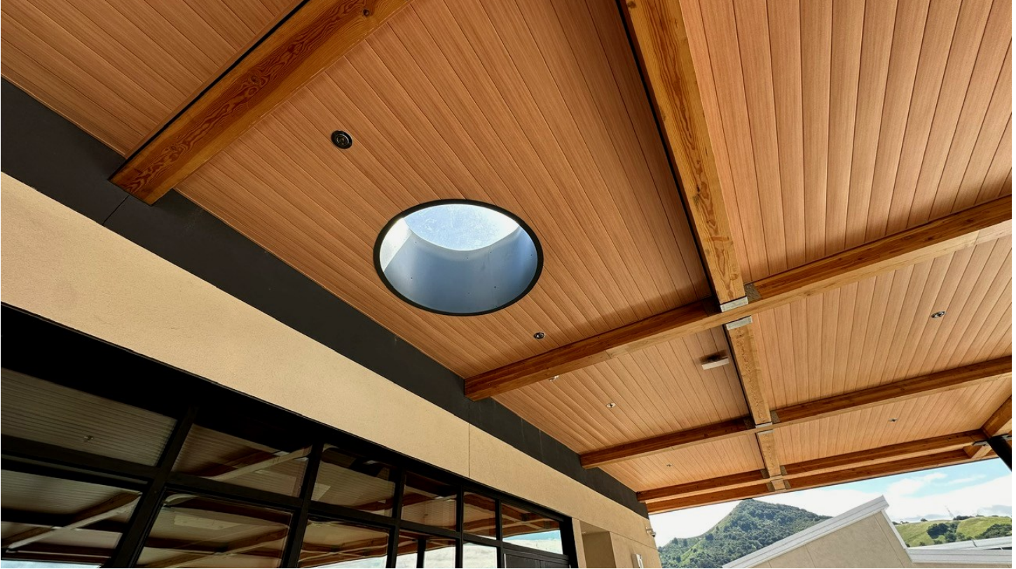
Skylight Drum Installation
