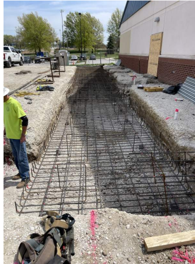
EPiC Elementary - Footing Prep
