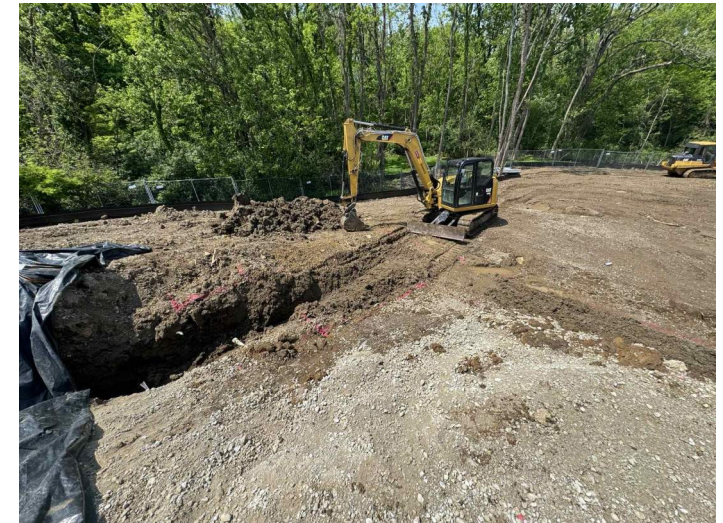
EPiC Elementary - Digging Footings
