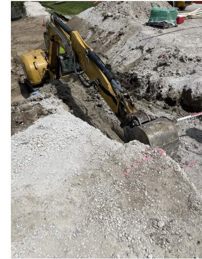
EPiC Elementary - Digging Footings
