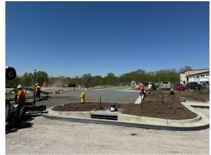
Pouring New Drive at North Entrance
