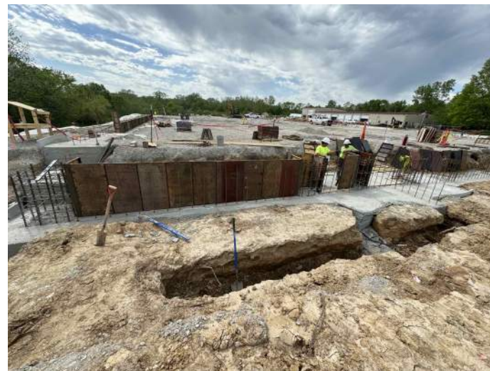
Footing at Southeast Corner of Building
