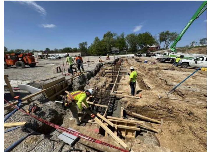
Footing at Southeast Corner of Building
