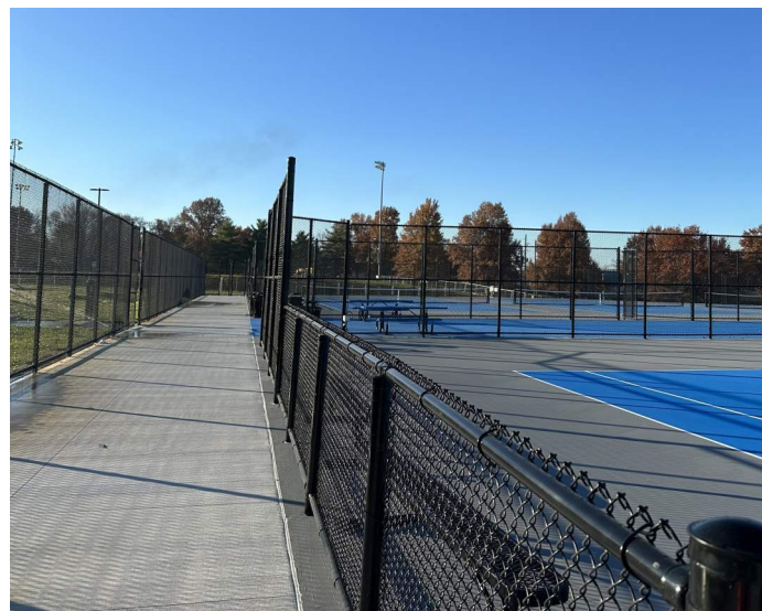
East Concourse Looking South
