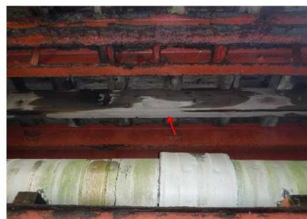
Photo 14: West side of Beam 12
