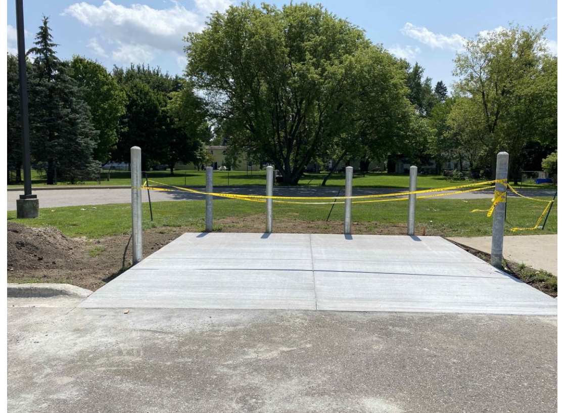
The new dumpster enclosure bollards have been installed, and concrete has been placed.
