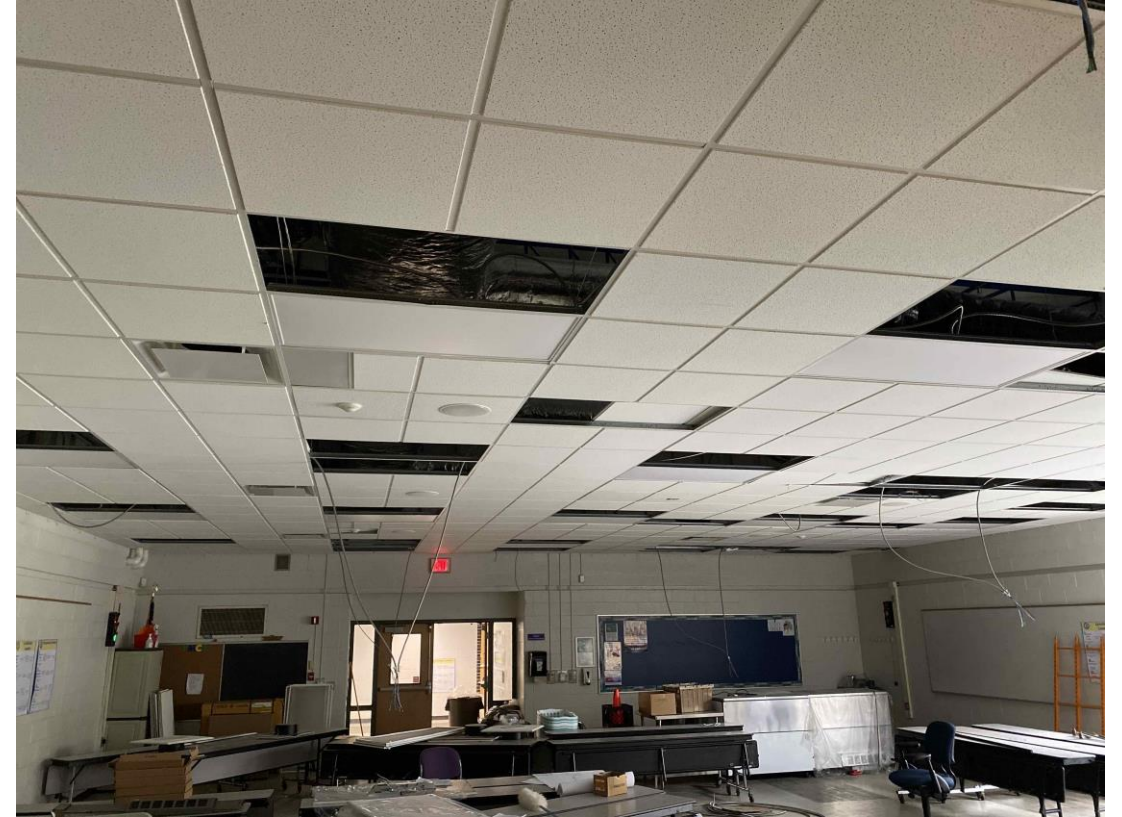
Ceiling tiles and lighting are currently being installed in the cafeteria.
