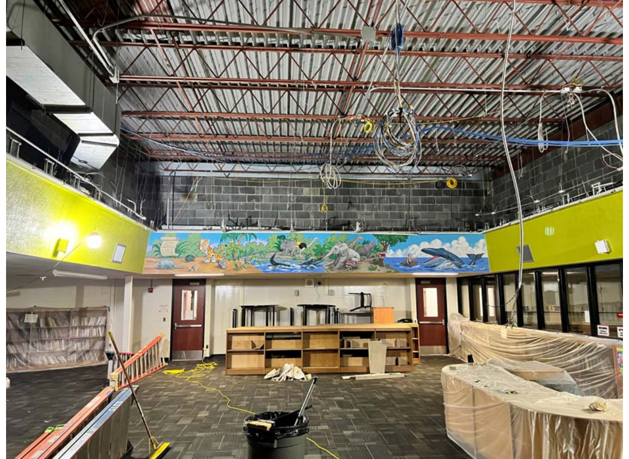
Existing ceiling grid removed, and new grid installation has begun in the media center
