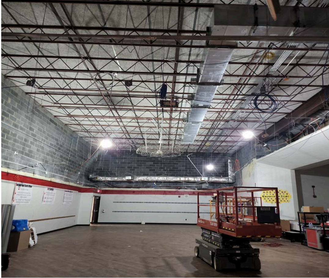
Existing cafeteria ceiling tiles have been removed in preparation for new ceiling height design
