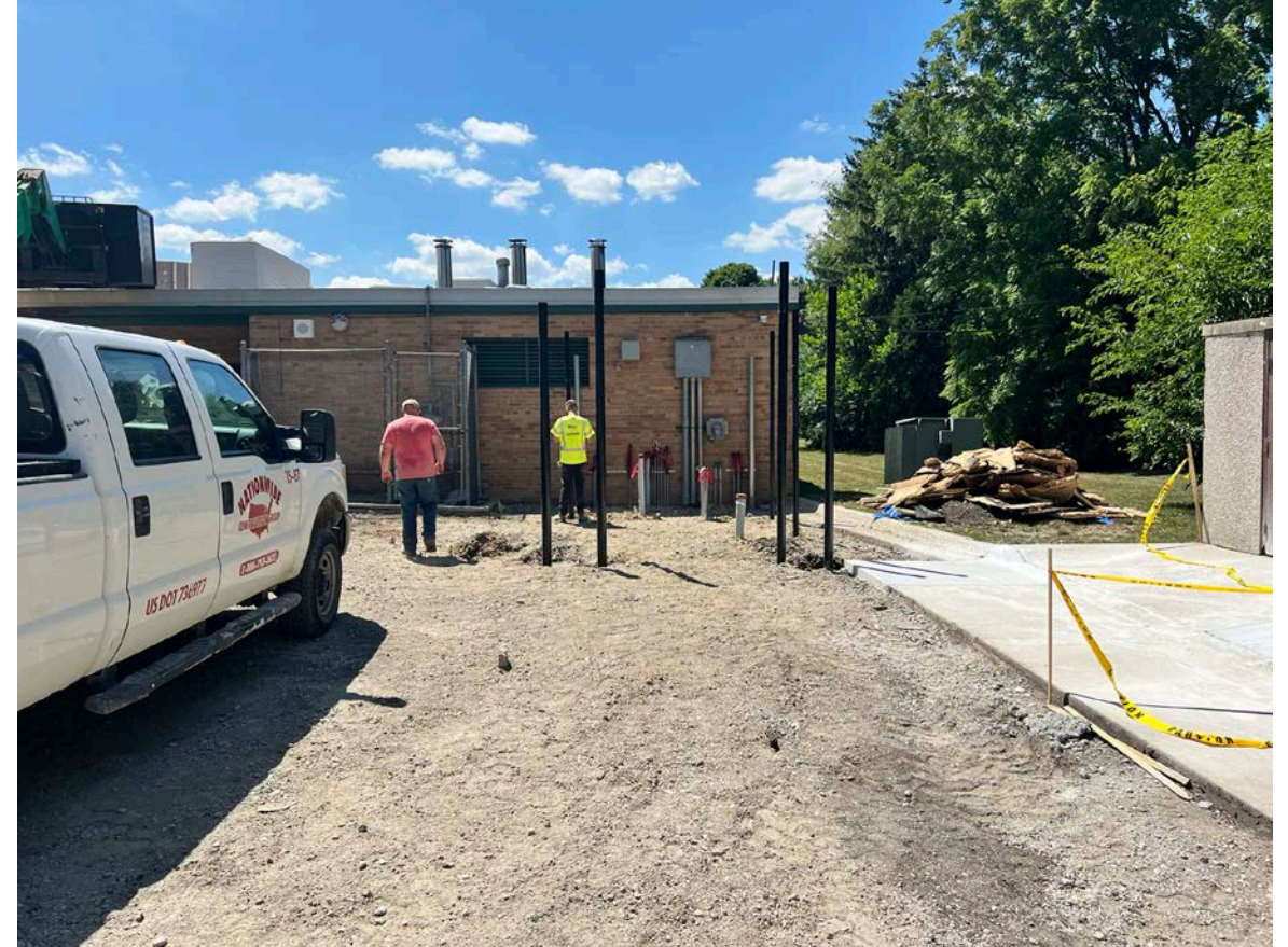
The new generator enclosure fence posts are being installed
