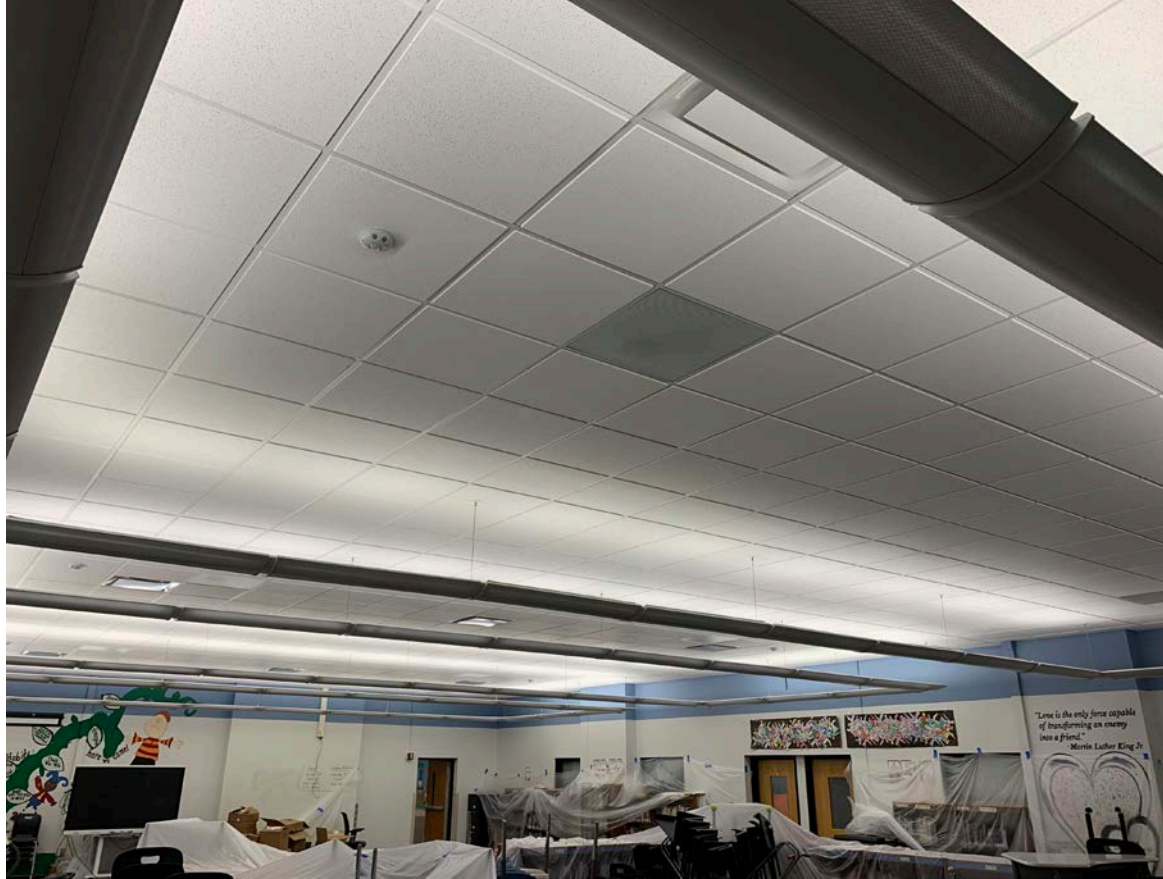
Selective new ceiling tiles are being replaced
