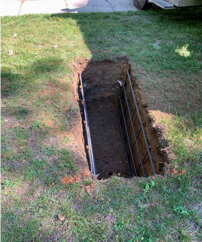
Sign foundation excavation was begun
