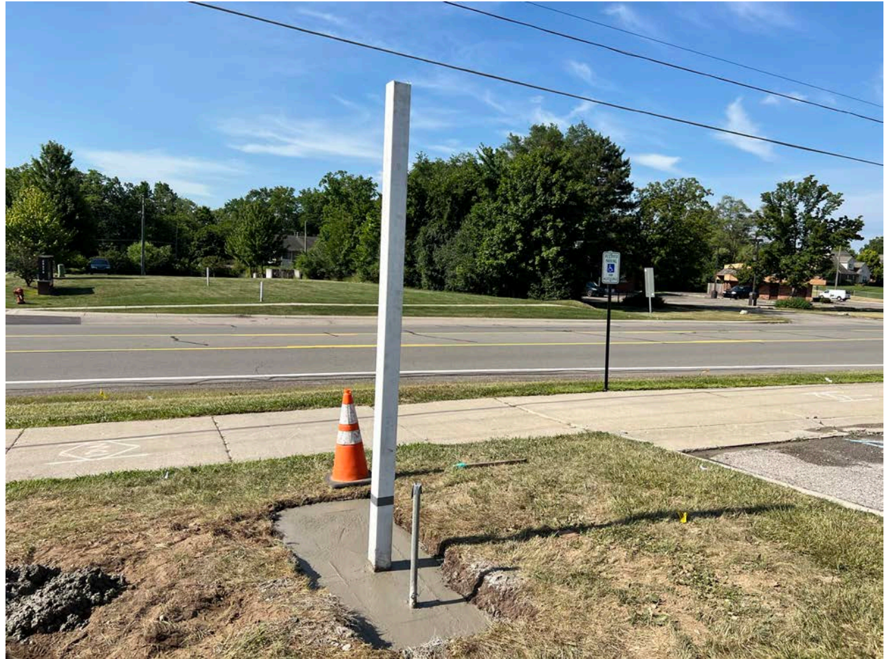
The concrete for the sign foundations has begun
