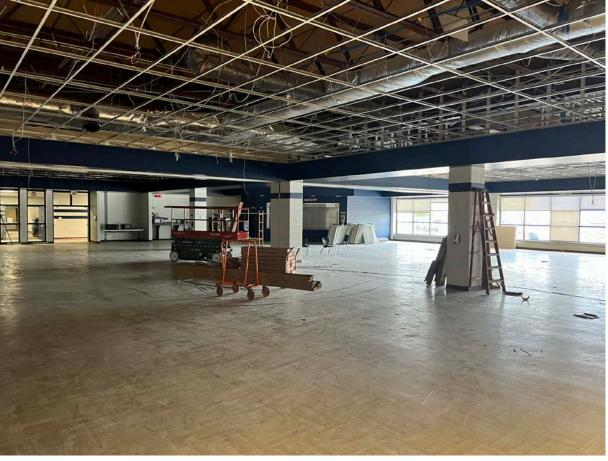
New ceiling grid has been installed in selective classrooms and the cafeteria. New ceiling tiles are starting to be cut and installed.
