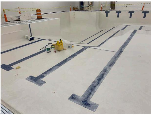
Pool re-grout work has been completed, and the pool is being prepped to be re-filled
