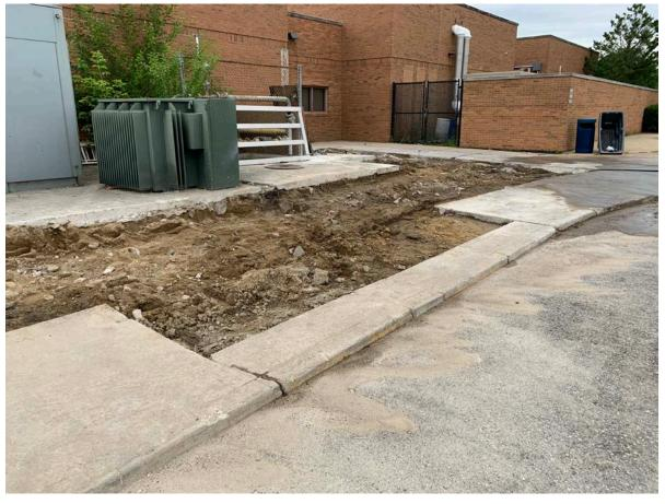
Demolition of exterior mechanical courtyard wall is complete. Area being prepped for installation of the new masonry wall.
