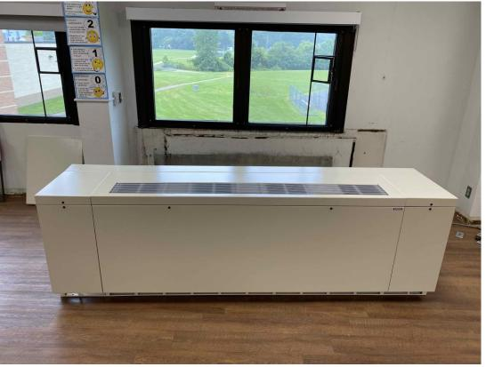
Existing classroom unit ventilators are being removed and new unit ventilators are being prepped for installation.
