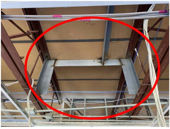
Media Center ductwork is currently being installed. The RTU structural steel support has been installed.
