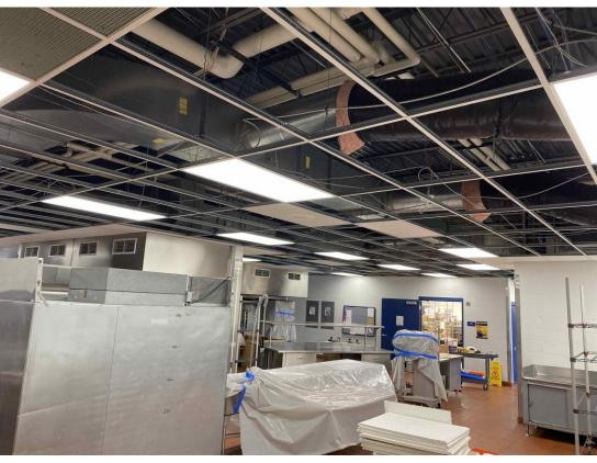
The new lighting and lighting controls are currently being installed in the Cafeteria and Kitchen
