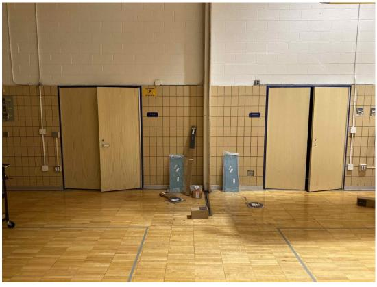
New interior doors have been installed and hardware is currently being installed
