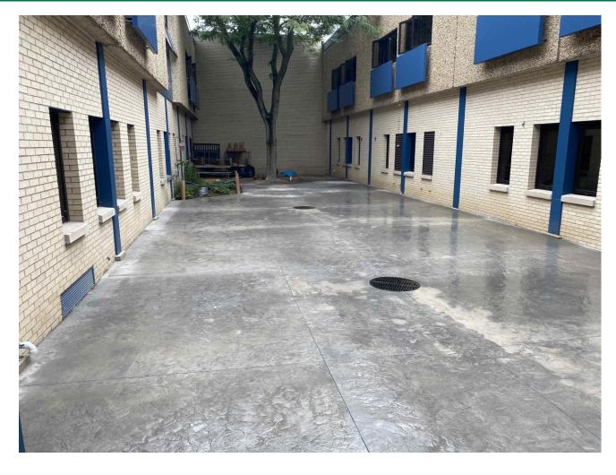
Courtyard concrete has been placed and stamped and drainage has been installed
