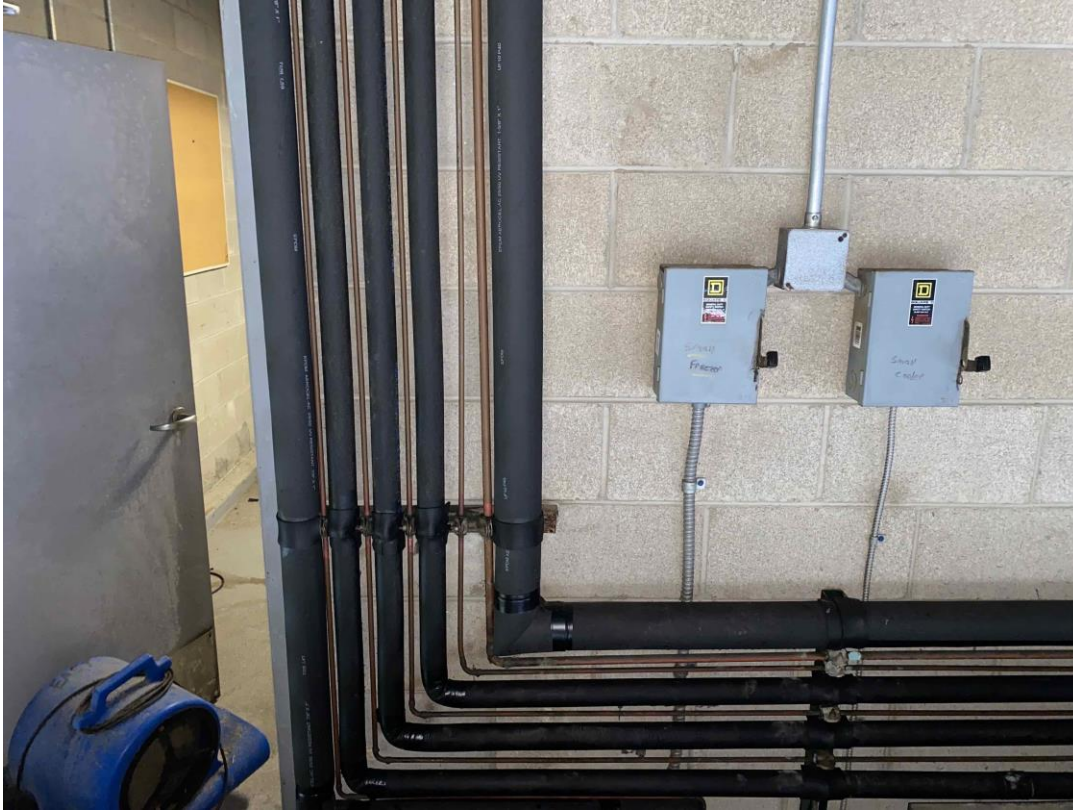
Refrigerant pipe in kitchen and mezzanine have been re-insulated
