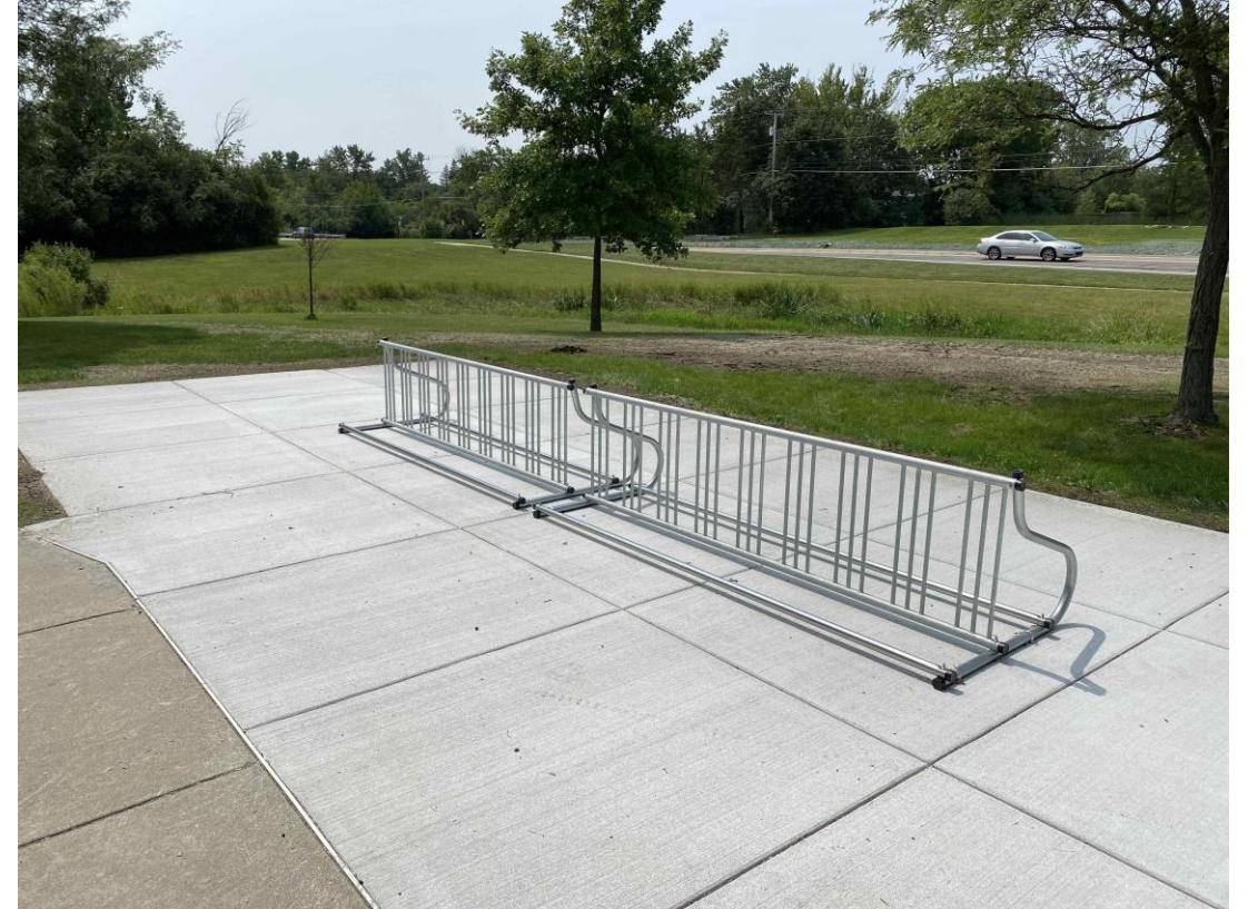
The new bike racks has been installed.
