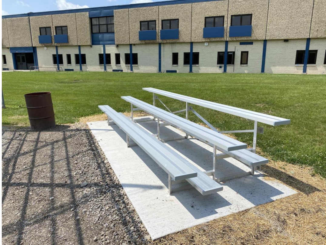
The new baseball field bleachers have been installed.
