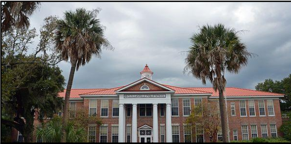
McClellanville Middle School (inactive)
