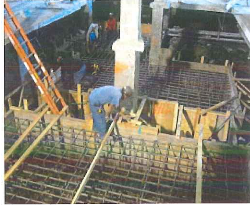
New Interior Structural Pile Cap
