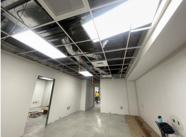
North Charleston HS Front Office – Building Improvement Project
