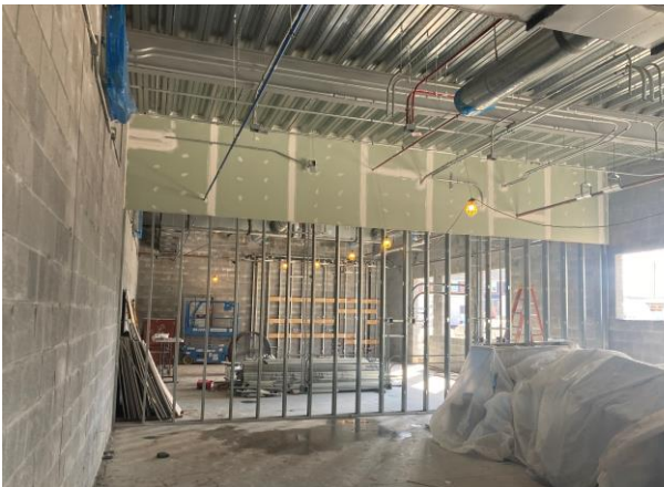
Typical Interior Classroom
