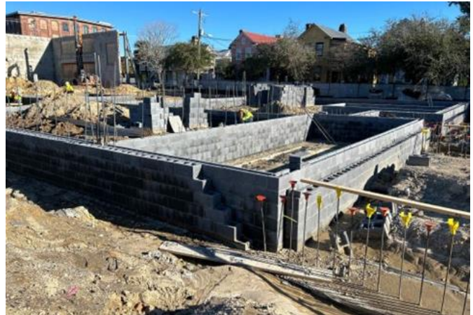
CMU Foundation Block and Underground Utilities
