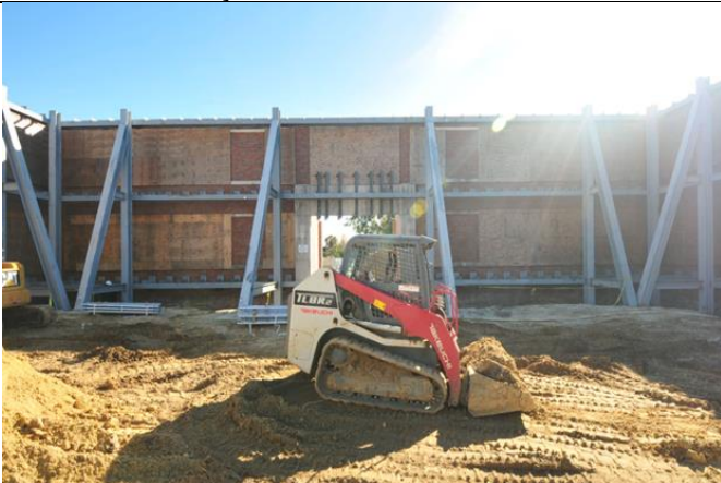
Entrance at Columbus Street – Temporary Bracing
