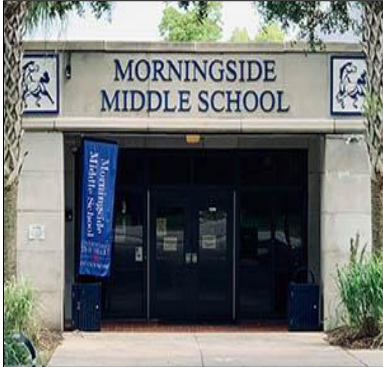
Front Facade Preserved at Morningside
