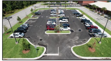
E.B. Ellington Parking Renovations
