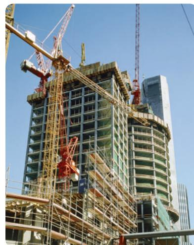
A typical tower crane can lift up to 18 metric tons of material at one time.
