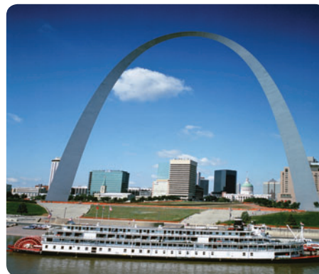
Gateway Arch in St. Louis is the tallest national monument in the United States. The shape of the arch is known as a catenary curve .
