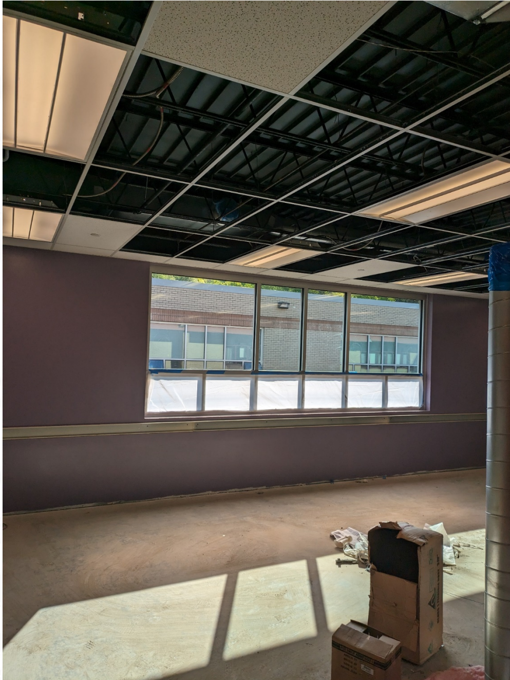
Accent Wall in Area B. Wallmold is being installed and wired.
