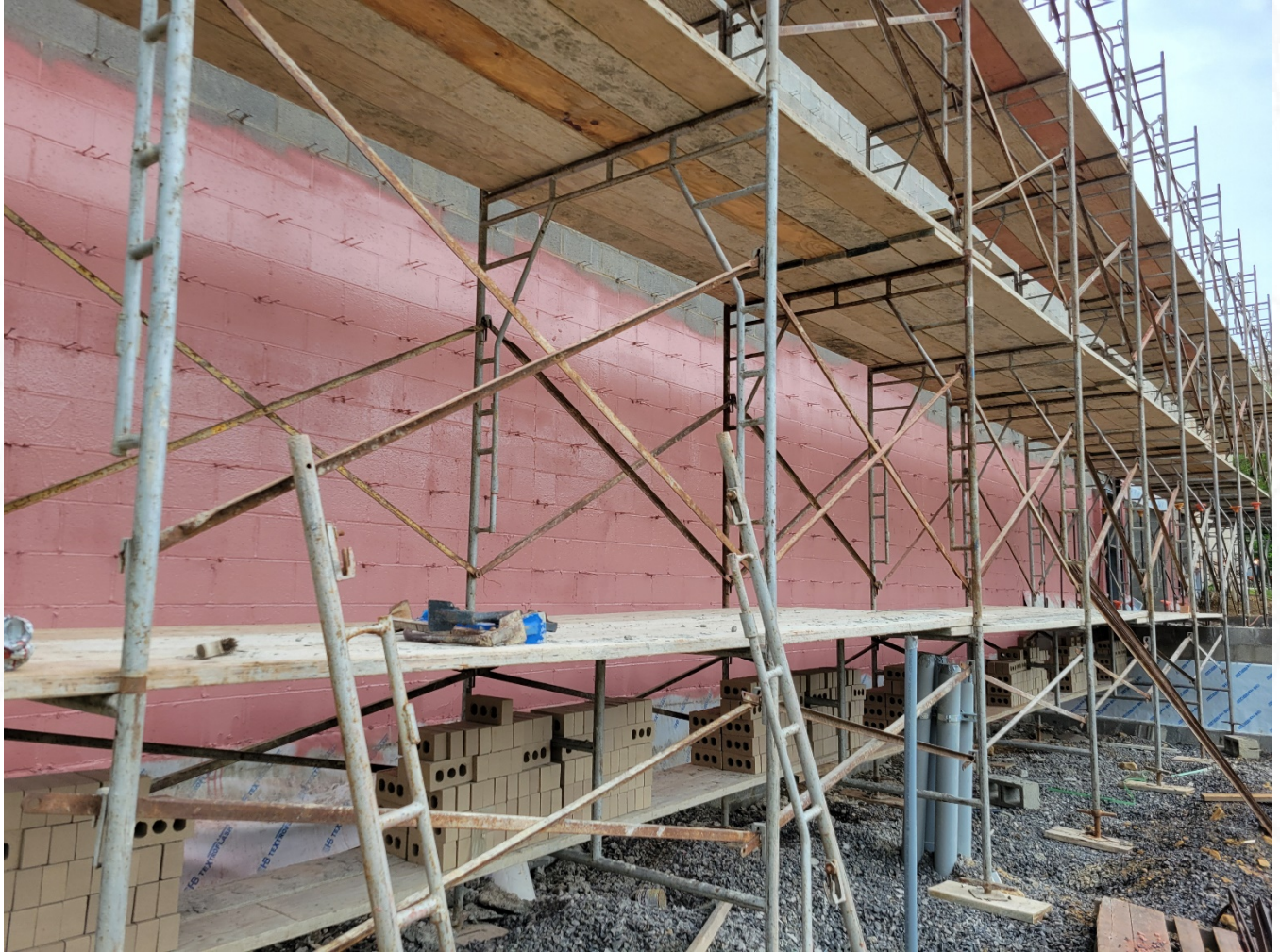
Air Barrier and brick ties in place, brick veneer staged for installaiton on south wall of cafeteria
