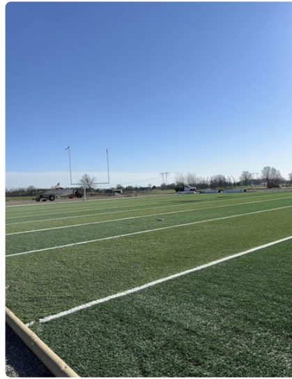
Turf Installation Underway
