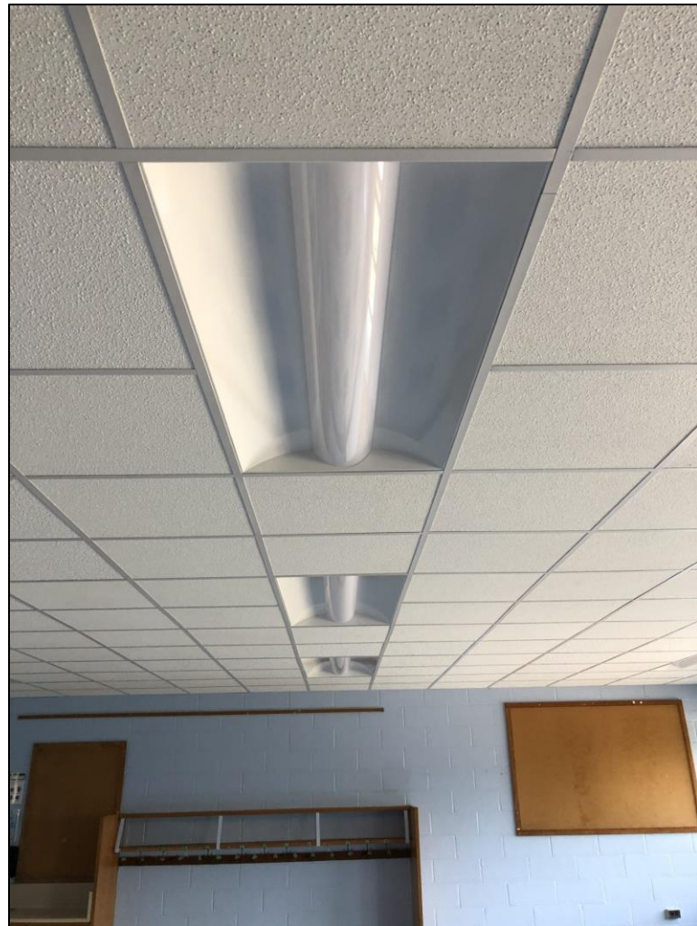
Ceilings in Manor & Harbor Elementary Schools
