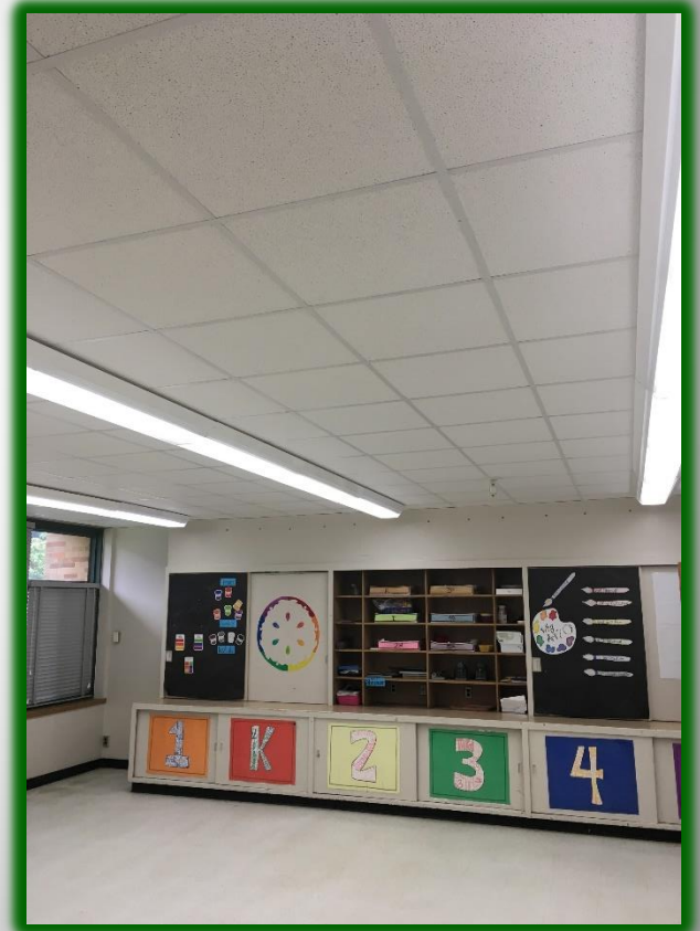
Ceiling Replacement A Wing
