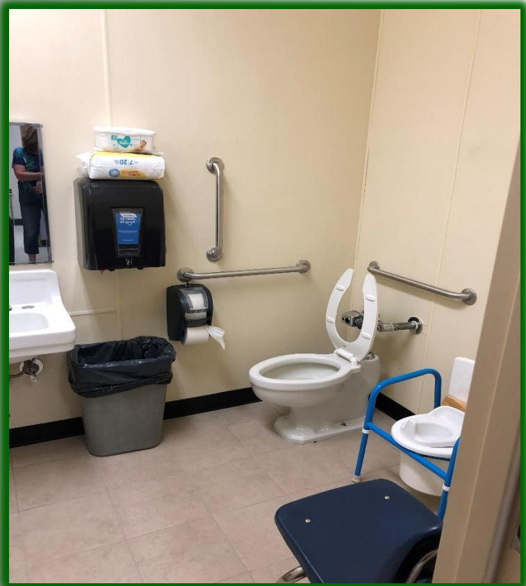
Handicap Bathroom Renovation
