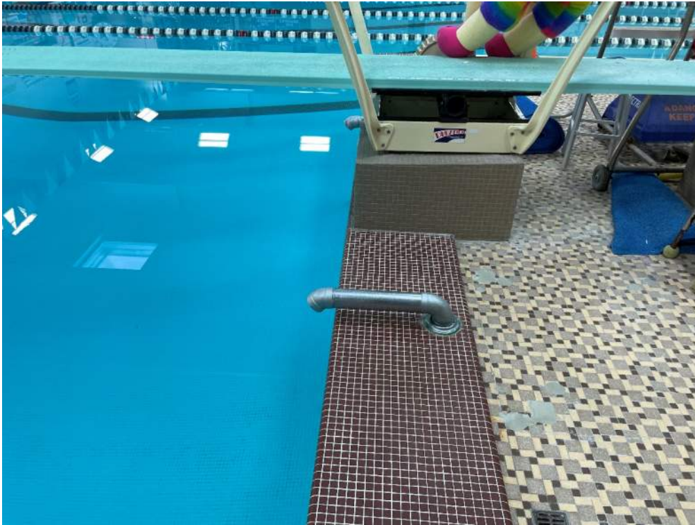
Pool Wall & Tile – Good Condition
