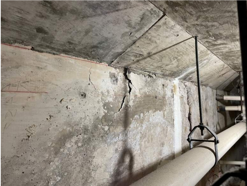
Large Spalling Area
