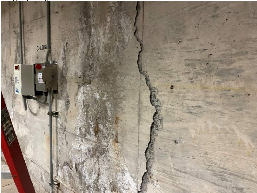
Large Spalling Area
