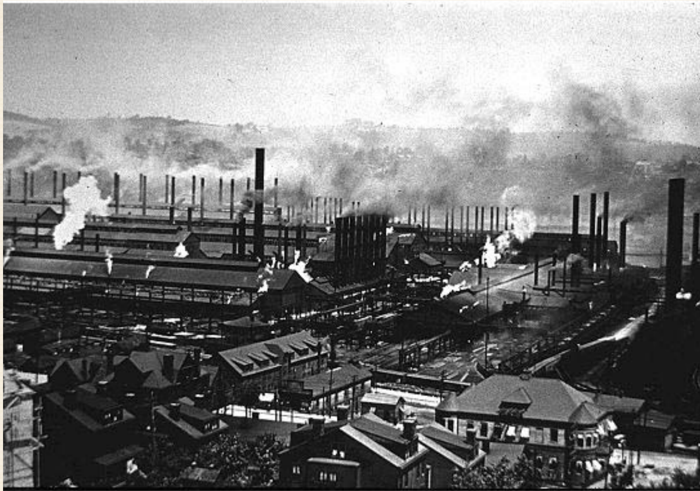
Homestead Steel Plant - near Pittsburgh, PA
