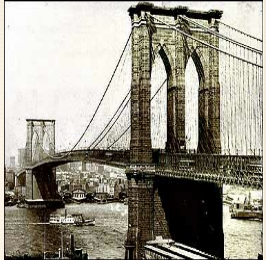
Brooklyn Bridge, 1883 Longest span 1,595 feet
