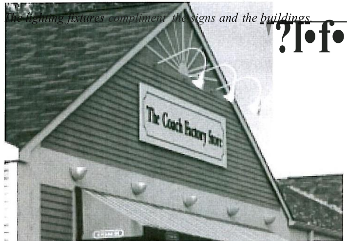
In both examples above and below the top-mounted light fixtures are well-located, aimed, and shielded so that only the sign is lit
