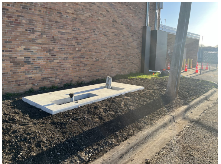
New conduits installed for rooftop air-handling unit; patching with concrete; concrete transformer pad (April 2024)
