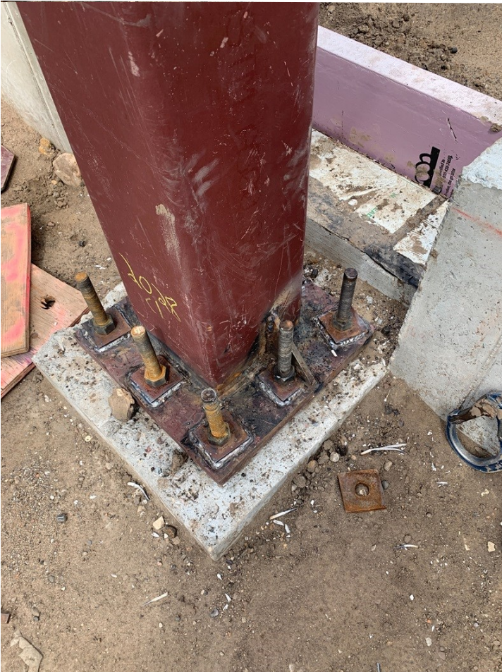
From top, left to right: Steel columns on north end of site; joists and beams; anchor bolts on steel column; steel looking west (April 2024)
