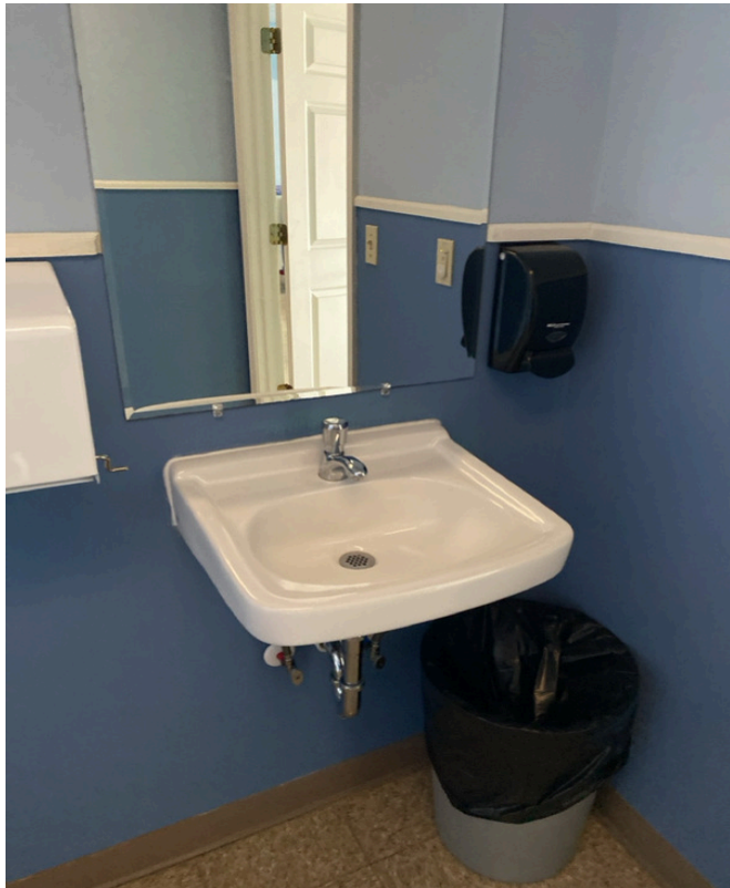
3/22/2024 - 1115-24 - Liberty Academy - 001909- Room 109-Restroom
