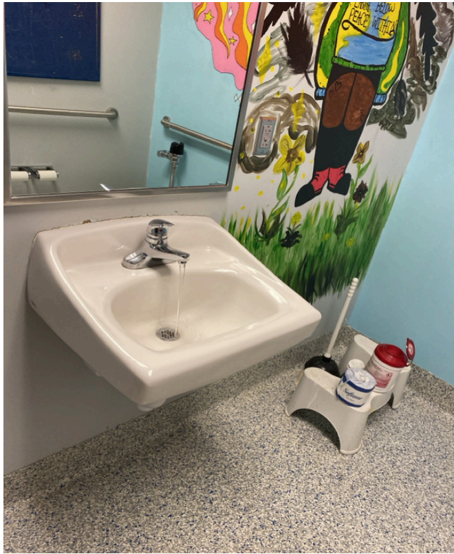
3/22/2024 - 1115-20 - Liberty Academy - 002226- By 206-Staff Restroom
