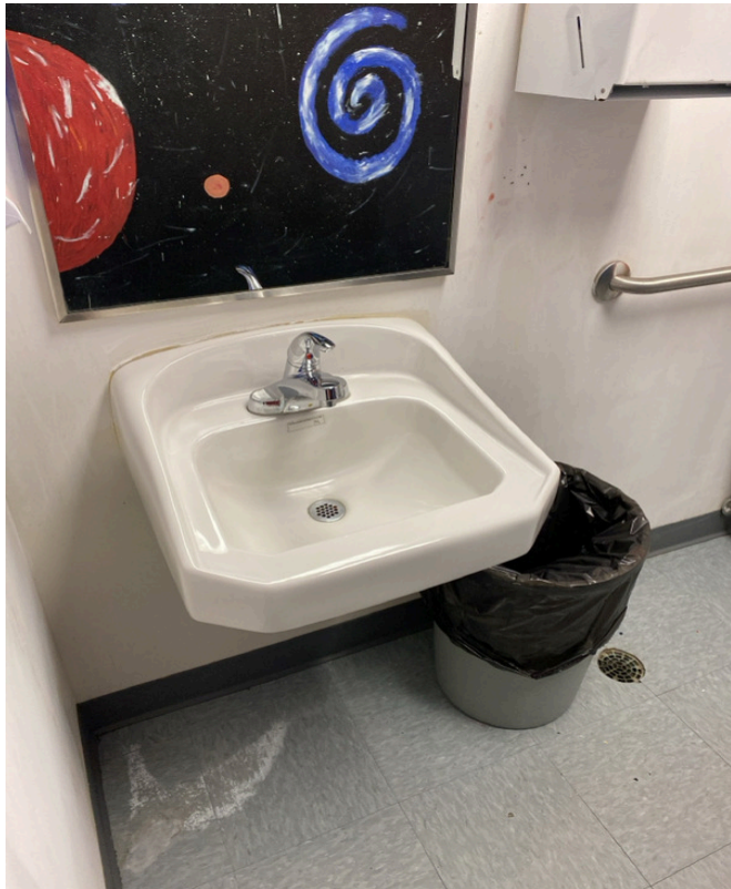
3/22/2024 - 1115-9 - Liberty Academy - 001920- 1st Floor-Staff Restroom
